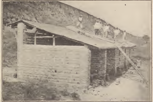
ROOFING THE MISSION STABLE
